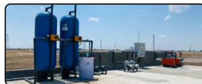
STP in Civil Work
