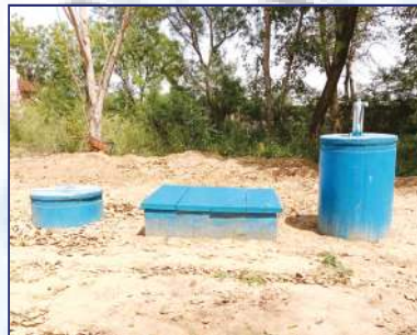
Injection Recharge Well Technology for Loose Area
