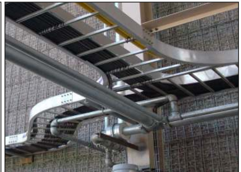
Cable Tray Installation
