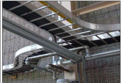
Cable Tray Installation
