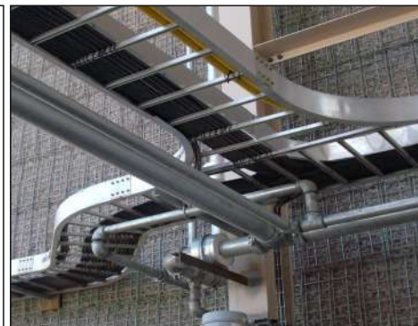
Cable Tray Installation
